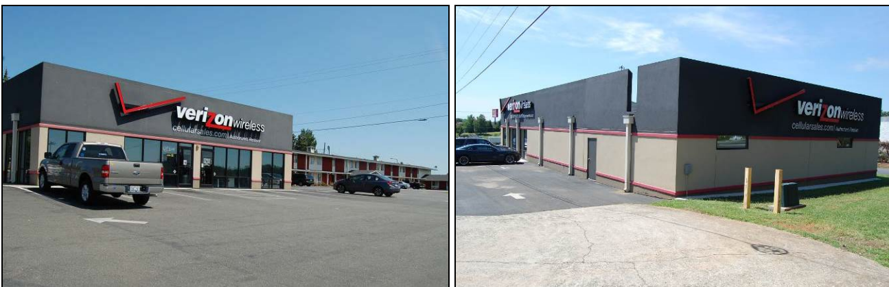
Figure 24. Verizon building looking northeast, at left, and southwest, at right
