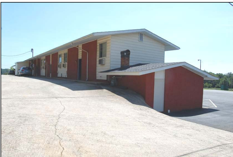
Figure 16. North elevation looking southeast
